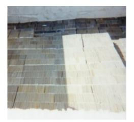
Each canister is filled by installing one 4-inch layer of media at a time. All of the modules in a layer should be placed in the same orientation, with all the ceramic plates parallel to each other. The following layer should be installed similarly, but rotated  $90^{\circ}$  so that the plates are perpendicular to the plates in the layer beneath it.
