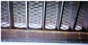
installed on a supporting structure which has as much open area as possible. A rectangular grid of metal bars spaced ~1 inch apart works well for MLM<sup>®</sup> modules, although smaller openings are needed if ceramic balls are used to fill gaps (See section 7, below)
