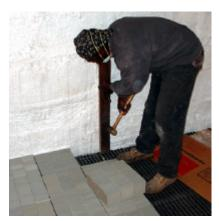
MLM<sup>®</sup> should not be installed until after the insulation along the inner walls of the canisters has been completed.
