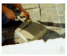
flat screwdriver at mid-height of the adhesive layer on the side of the module.
